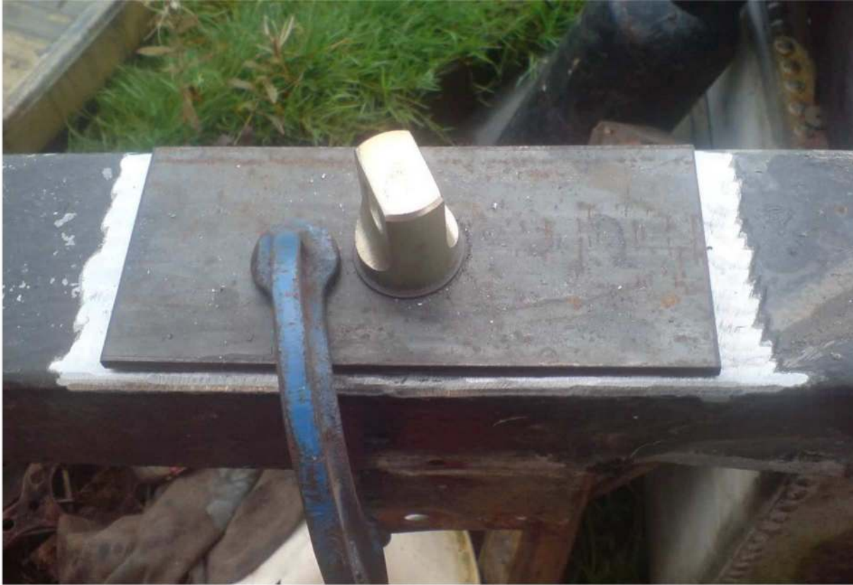
Stick welding FTW 🤔
